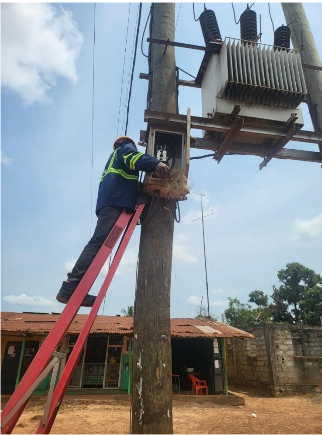
A technician removes a bird nest from a breaker
