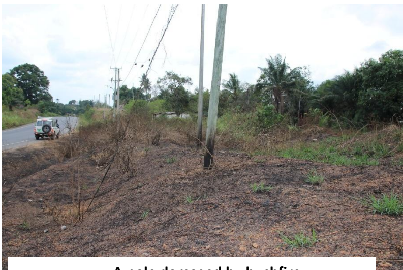
A pole damaged by bushfire
