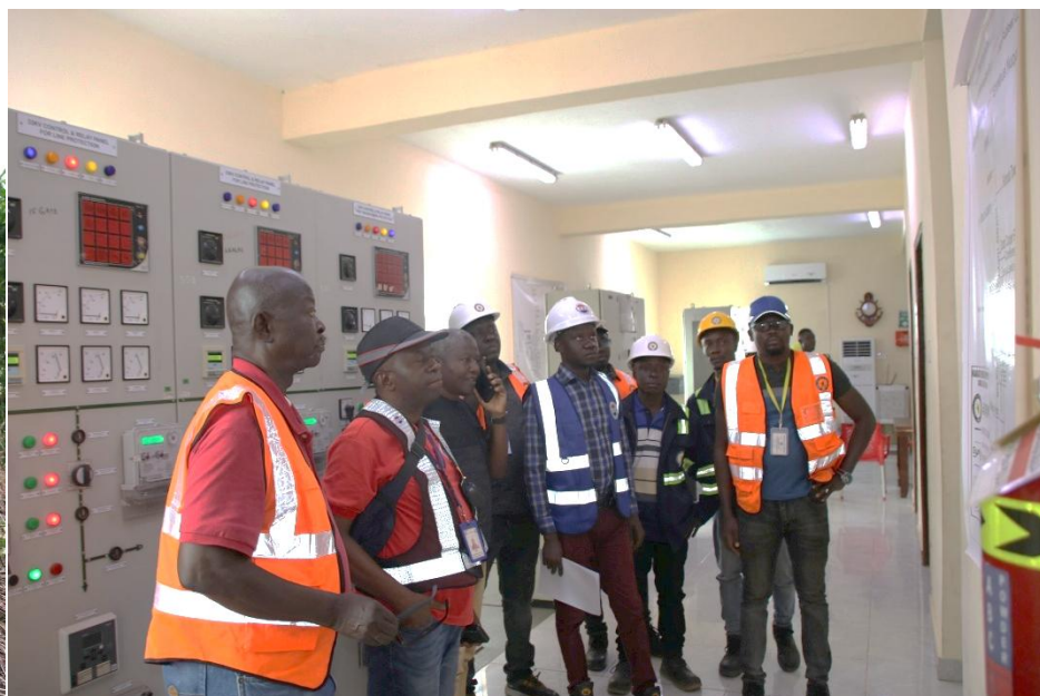
The team reviews the substation diagram
