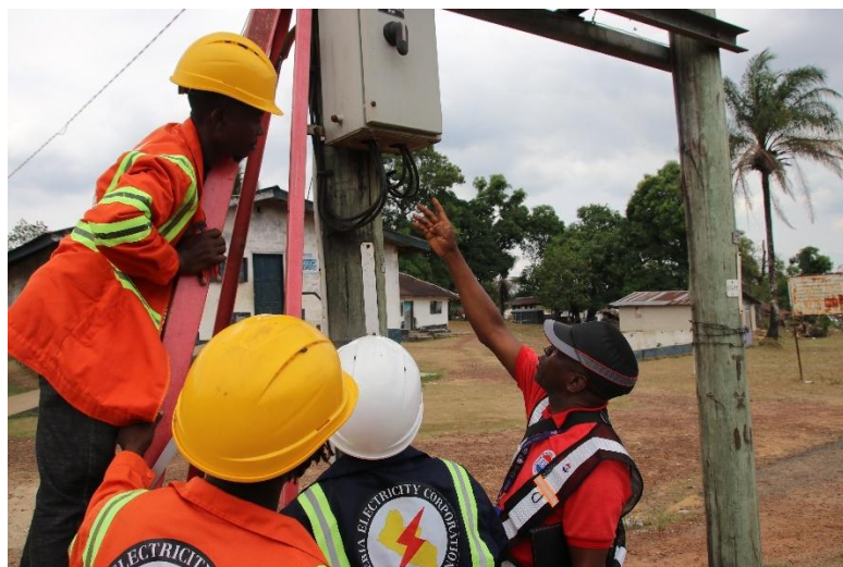
The team inspects a breaker with bird nest
